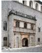
ND.I, Portalaltane, westl. Fassade, DE001382, BSV
