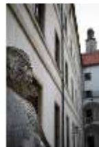
ND.I, Innenhof, Ostfassade, DI027419, BSV
