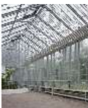
NyEi.II, Eisernes Haus, DI001516, BSV
