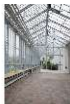
NyEi.II, Eisernes Haus, DI001515, BSV
