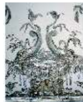
NyAm.II, Blaues Kabinett, R.3, Deckenstuck, Detail, DE004547, BSV
