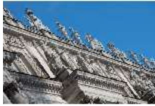
HchNS.I, Westfassade (Detail), DI018949, BSV
