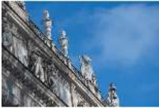
HchNS.I, Westfassade (Detail), DI018948, BSV
