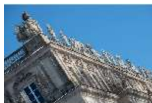
HchNS.I, Westfassade (Detail), DI018946, BSV
