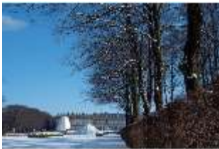
HchNS.V, "Parterre de Latone", Westfassade, DI018901, BSV
