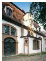
Ell.I, Reithalle, Ostfassade, DE003107, BSV-
