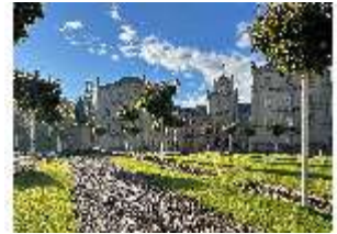
CoE.I, Hauptfassade, DI020875, BSV-
