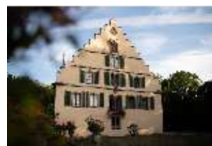
CoR.I, Nordfassade, DI025444, BSV-
