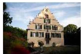
CoR.I, Nordfassade, DI025445, BSV-
