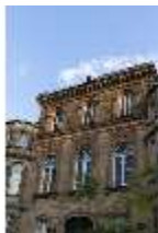
BayFa.I, Nordfassade (Detail), DI017167, BSV-
