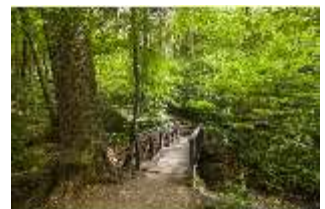
BayFa.V, Brücke, DI002612, BSV
