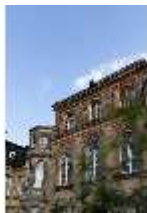
BayFa.I, Nordfassade (Detail), DI017166, BSV-
