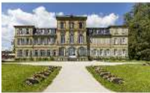
BayFa.I, Südfassade, DI002641, BSV
