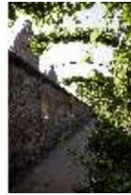
AschPomp.V, Laubengang (sog. Kapuzinergang), DI015031, BSV-
